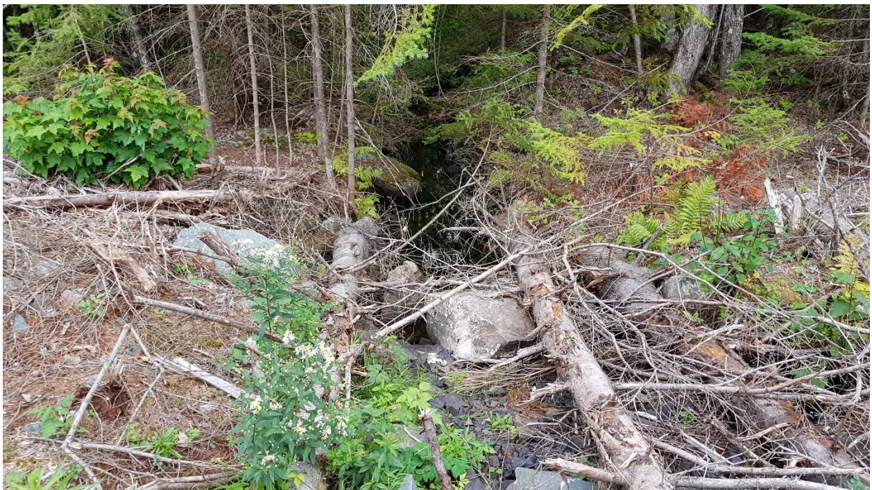
Photo 6. Area 4D – Looking downstream from the culvert above. A small current emanates from the embankment fill several metres downgradient.
