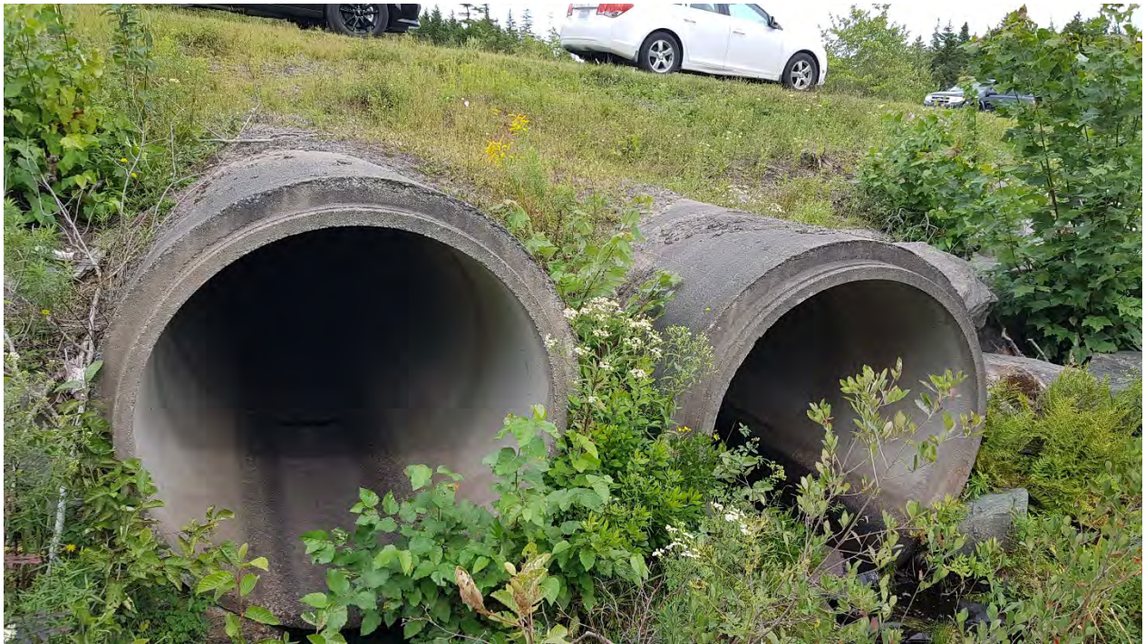
Photo 35. Mitchell Brook downgradient of Area 1E –Two large culverts (Culvert 2 in Figure 2) at Mitchell Brook where it crossed the highway.
