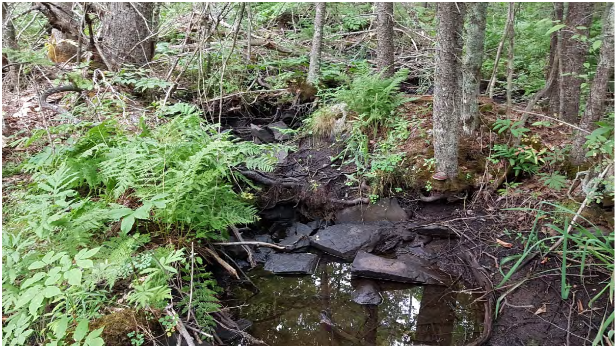
Photo 4. Area 4D – A steep intermittent stream flows from Area 1E via Culvert 1. There are signs of seasonal high-volume flow. The flow infiltrated into the ground before reaching the wetland.
