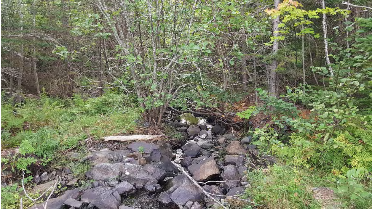
Photo 7. Area 4B – Looking downstream from Culvert 3, the drainage to Area 4B is intermittent in summer, frequently disappearing below ground but flowing permanently in sections.
